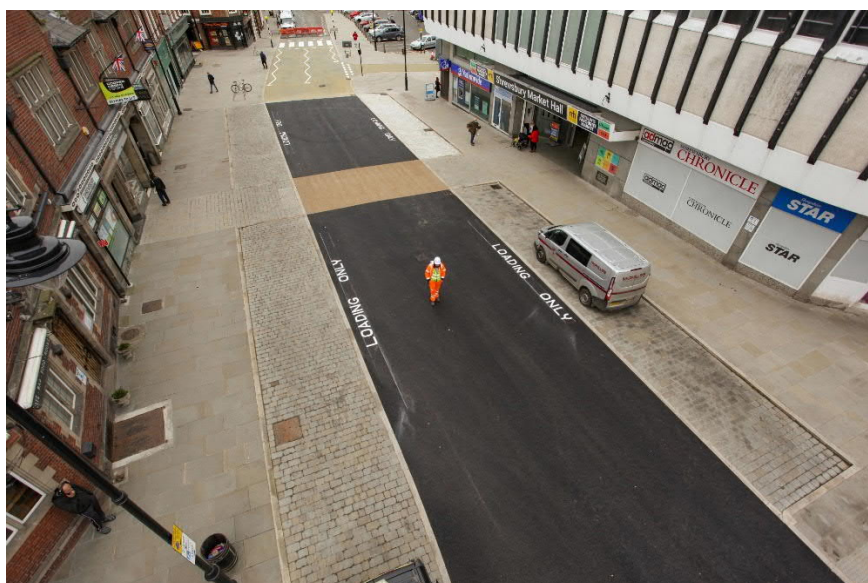
Bellstone, April 2021, awaiting installation of street furniture
