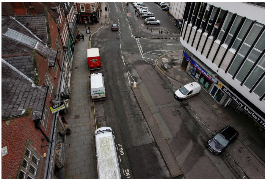
Bellstone, before construction works, February 2020, view North West towards Barker Street
