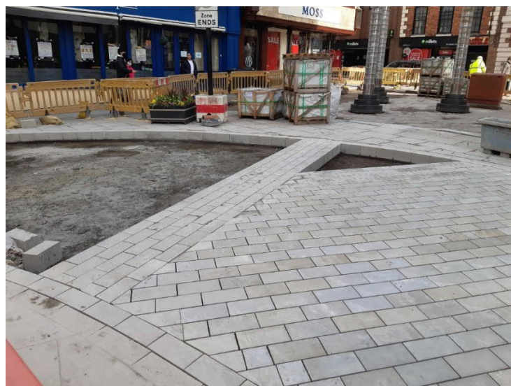
Mardol – Claremont Street corner, showing carriageway construction using stone setts
